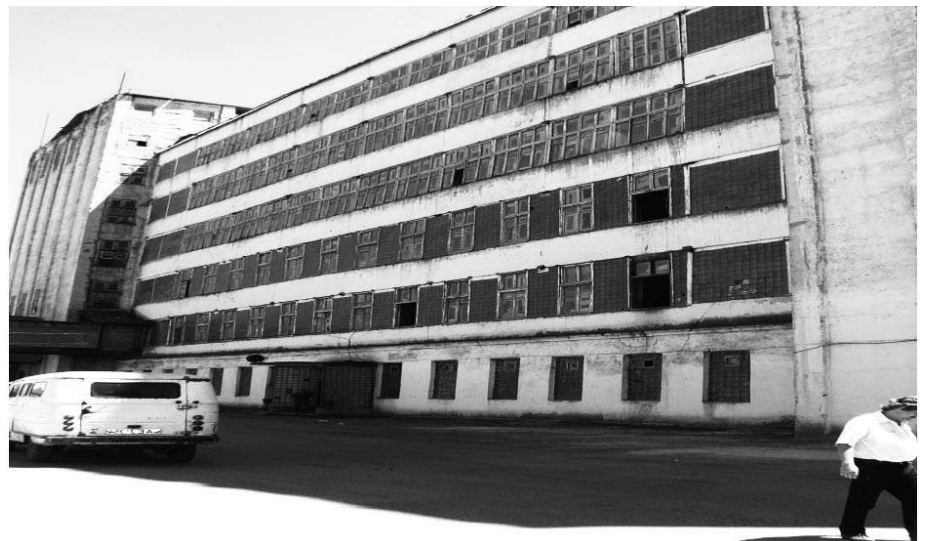
This flour mill's infrastructure may have needed updating but its pest management program was very modern.
