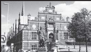
The Børsen (Royal Stock Exchange Building and Conference Center)
