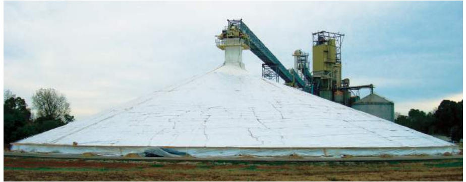
Circle Pile; temporary storage of 900,000 bushels of corn.
