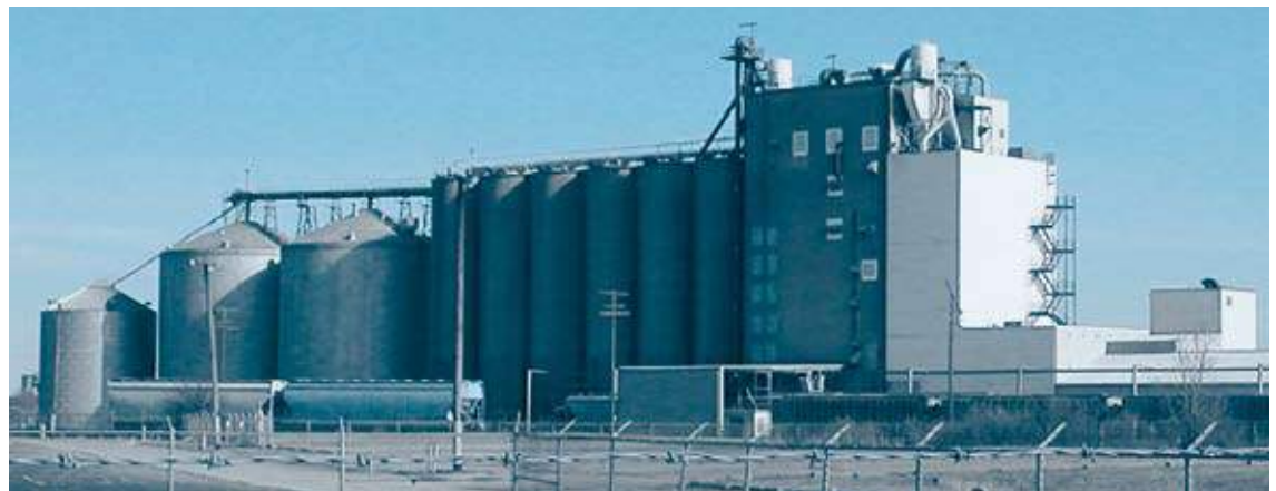
Flour mill, grain storage silos, railcars all need different fumigation technology.
